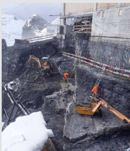
Baugrubenaushub Birg Tal
